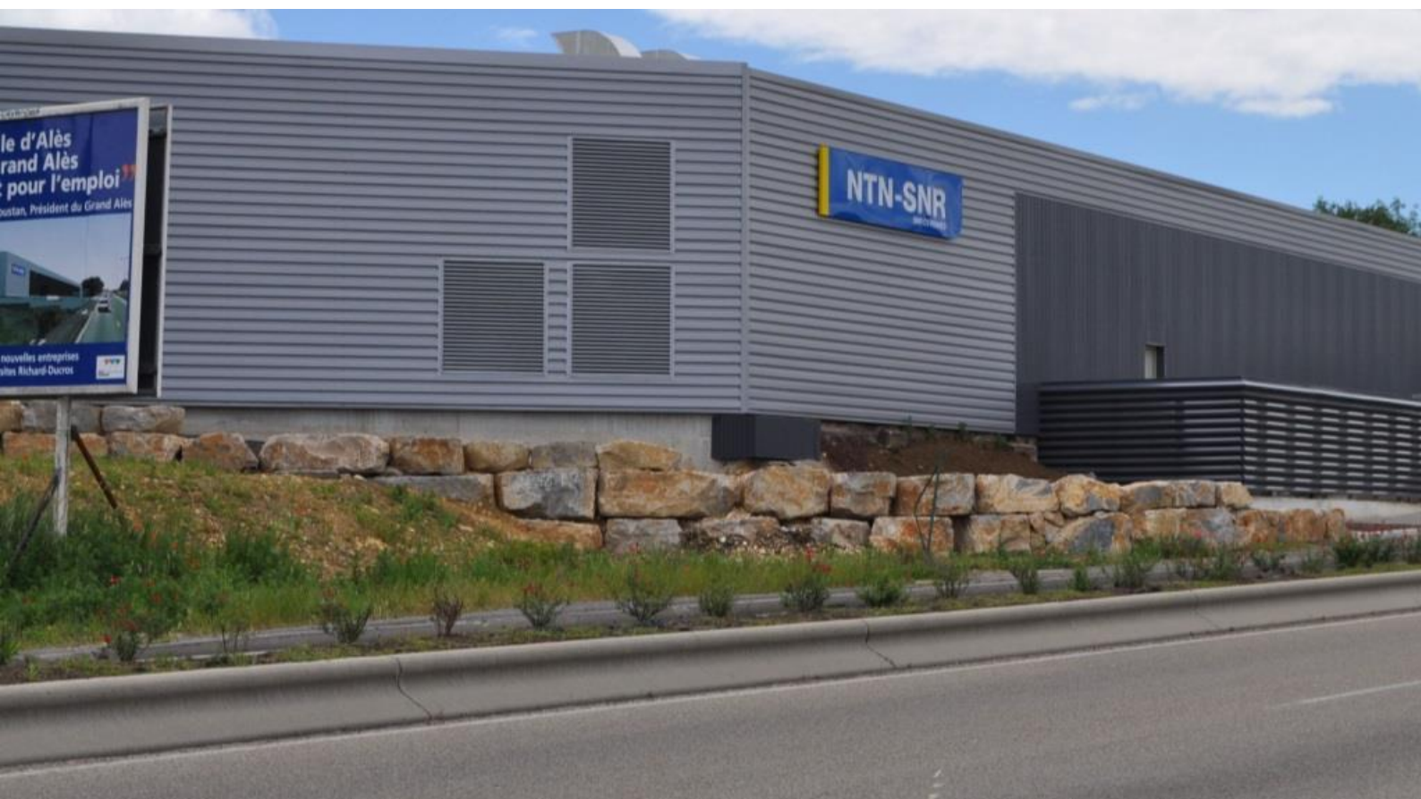
The Croupillac factory, a Factory of the Future integrated into its urban environment
