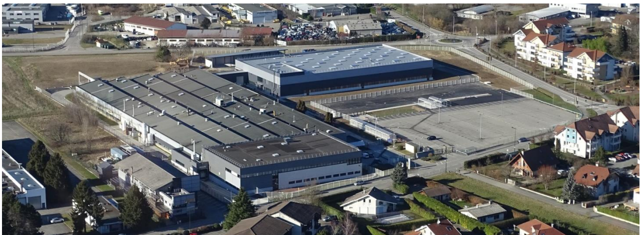
The Argonay factory and its new building, the “Factory of the Future”
