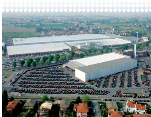
Head office of SAME DEUTZ-FAHR at Treviglio (Italy)
