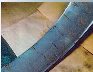
Downtime caused rust
